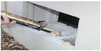
3. APPLY EXTERIOR GRADE CAULK AROUND WALL SIDE OF TRIM FLANGE (CLEAR CAULK RECOMMENDED) AND SLIDE FLOOD VENT INTO THE OPENING.
