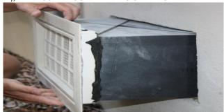
2. APPLY HEAVY DUTY ADHESIVE TO BOTTOM AND SIDES OF FLOOD OPENING
